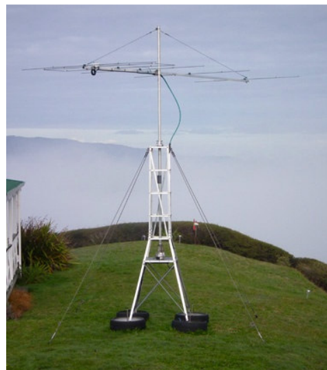
Overview of tower using only 2 sections supporting large 6m Yagi
